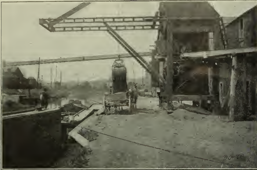
FIG. 2. UNLOADING COAL FROM THE CANAL
